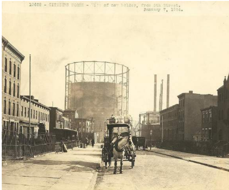
Figure 3. Citizens Manufactured Gas Plant 1924.
